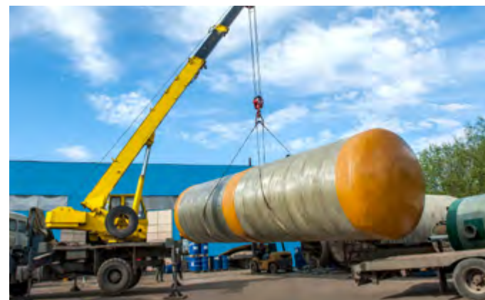
Loading of a Fiberglass Tank
